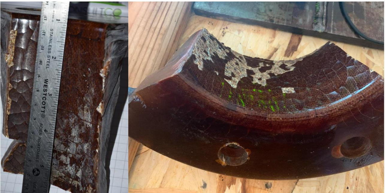
Figure 4. Inside surface condition and corrosion of the FRP
